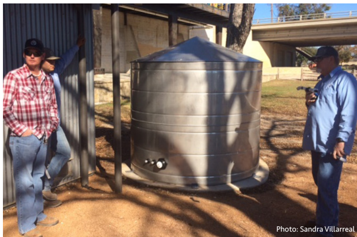
Installation of a rainwater harvesting system in a central park in San Angelo, TX.
