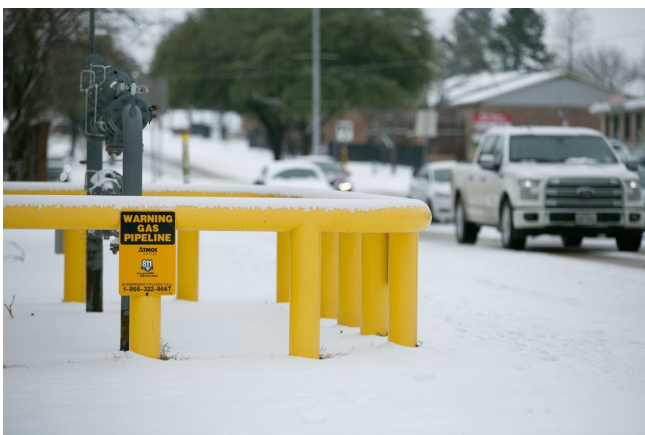
Fig. 21. Cold weather caused natural gas pipeline compressors to be inoperable. Source: Wall Street Journal (55)
