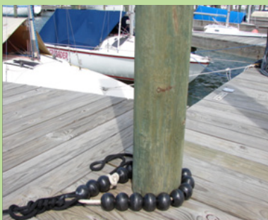
Tide risers enable moorings to rise when sea levels are elevated.
