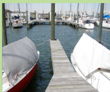
Floating docks break away from the pier during storm surge events, preventing the docks from pulling boats away.
