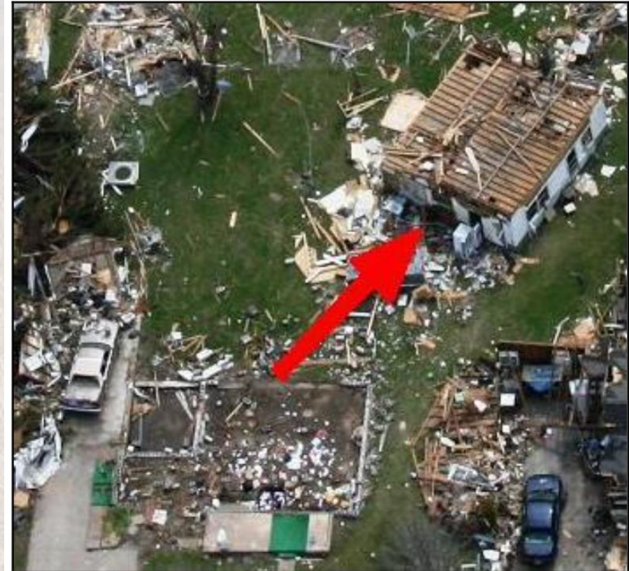
Figure 4. Example showing a home that was “swept clean” from its foundation that was rated EF-2 based the removal of its roof. Note vehicle remained within the destroyed garage.
