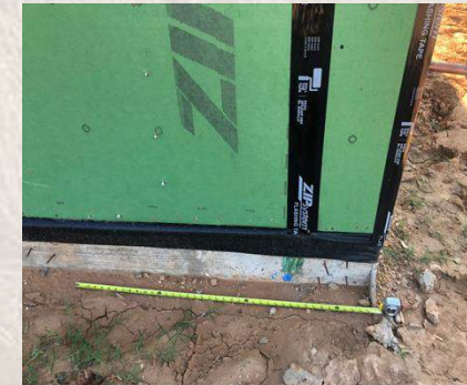
Bolts +rigid sheathing overlapping Bottom Plate
