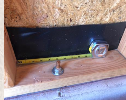
Bolts with nuts and standard washers
