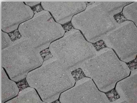
Figure 13: Example of permeable pavement (courtesy of Miami Group Sierra Club).
