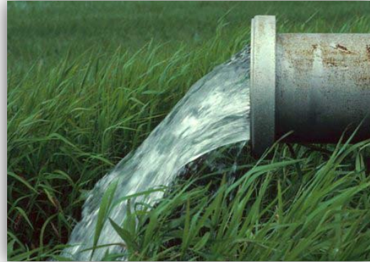
Figure 11: Example of a water pipeline (courtesy of San Francisco News).
