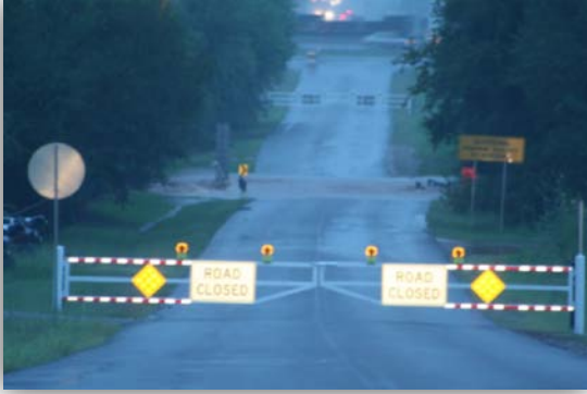
Figure 8: Low water crossing in Moore, Oklahoma. City officials installed gates to keep people from crossing the creek when it floods (courtesy of Gayland Kitch).
