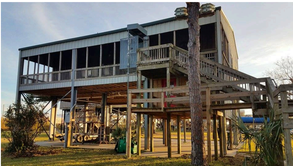
Figure 14: House on stilts in far southeast Louisiana, seen during Dr. Keim's tour.
