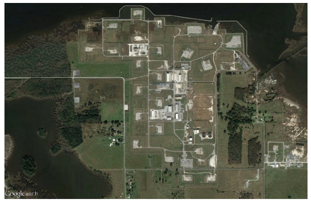
Figure 15: West Hackberry Strategic Petroleum Reserve site.
