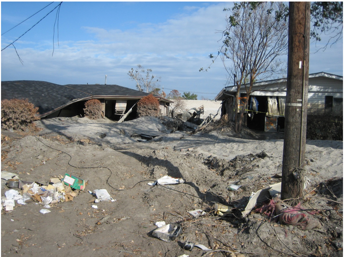
Figure 2. Sandy deposits near one of the breaches on the London Avenue Canal on Pratt Street. Image credit goes to Infrogmation and it can be found at https://commons.wikimedia.org/wiki/File:HousesPrattBehindLondonAvBreech.jpg .
